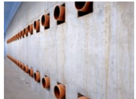
Temperature regulation using air exchange in Thüringen, Austria
