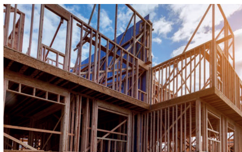
Framing wood construction (sample)
