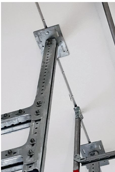
Fixing of installation system with MQM wing nut and hexagon bolt
