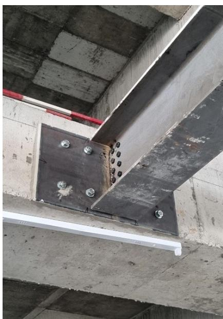
c) Detail of steel to concrete connection
