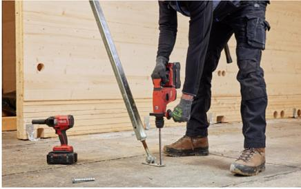
a) Drilling holes with a Rotary hammer
