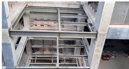
b) The steel frames are connected by anchors to the reinforced concrete structure
