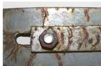
c) Corrosion of a steel bracket in an indoor swimming pool
