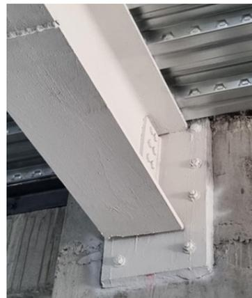
Fig. 6.11: Baseplate connection using group of anchors (4x2)
