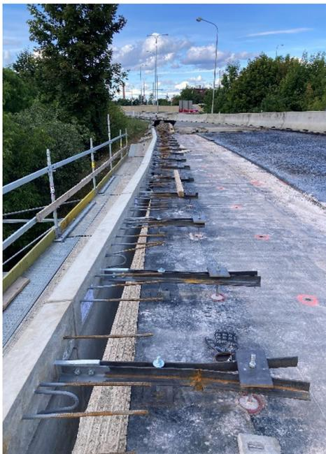
a) Steel cantilevers fixed by Hilti rods and RE 500V4
