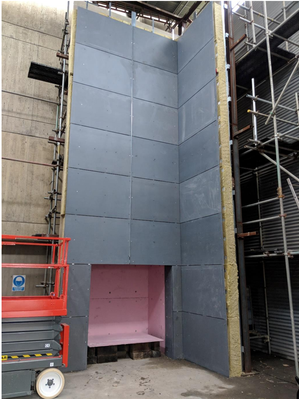
Figure 1 – Cladding system installation, pre-test.
