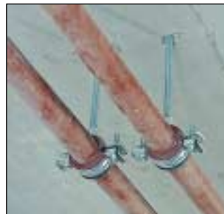
Multiple-pipe suspension made with anchors and threaded rods
