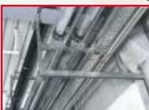
MQ system: – U-frame – Multiple pipe fastenings
