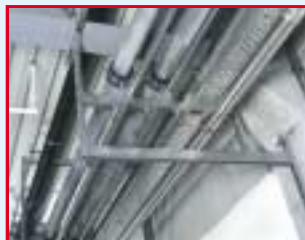
MQ system: – Bracket * – Channel structure * – MQW-S2 angle * * (Recognised by VdS)
