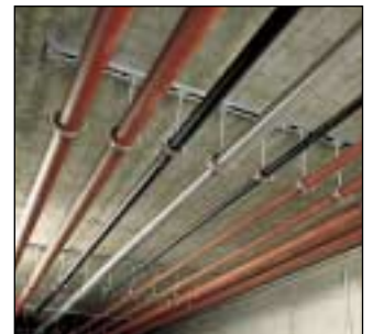
Multiple-pipe suspension made using an installation channel
