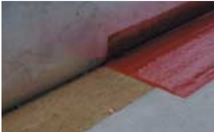
① Joints between floors and outer walls (facades)
